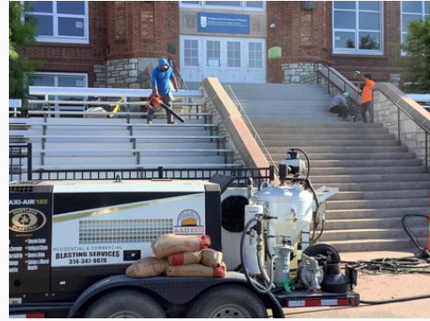
MSHS - New stair coating being installed.
